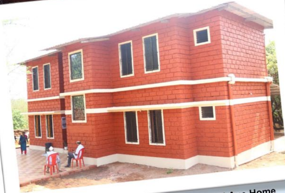
New building of Old Age Home
