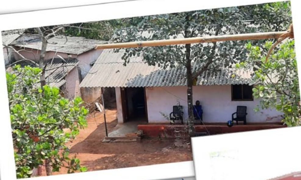
Old building of Old Age Home
