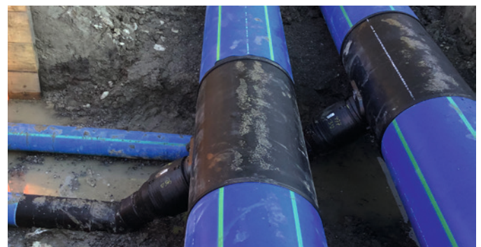
Safe and efficient: Factory-fabricated T-pieces can be used to create branches in the trench simply, quickly and reliably.
