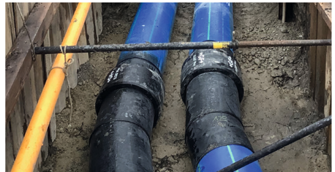
Problem-free and economical: Fixed point connections with ELGEF Plus couplers.
