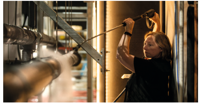
With a hard outer jacket and sealing lip, the corrosion-free COOL-FIT system can be easily power washed.
