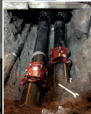
Installation company Van Kaam B.V. on site. Two MULTI/JOINTS® 3000 Plus, size DN300, were installed.
